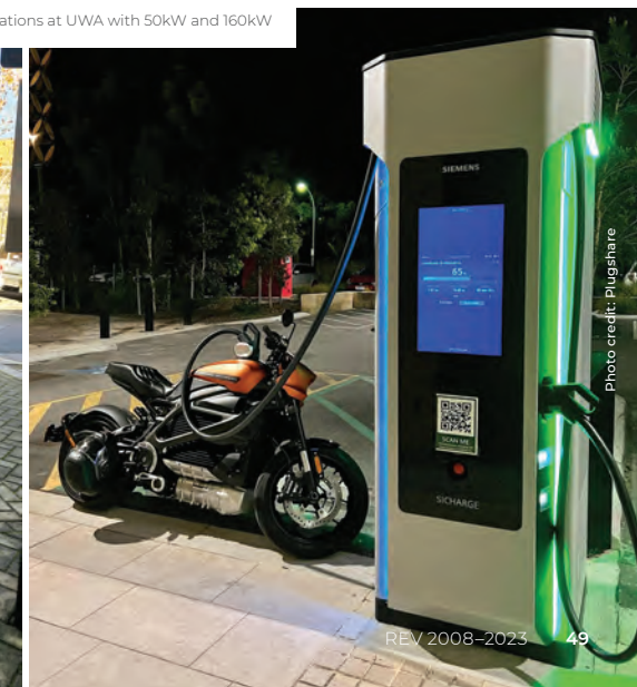
DC stations at UWA with 50kW and 160kW
